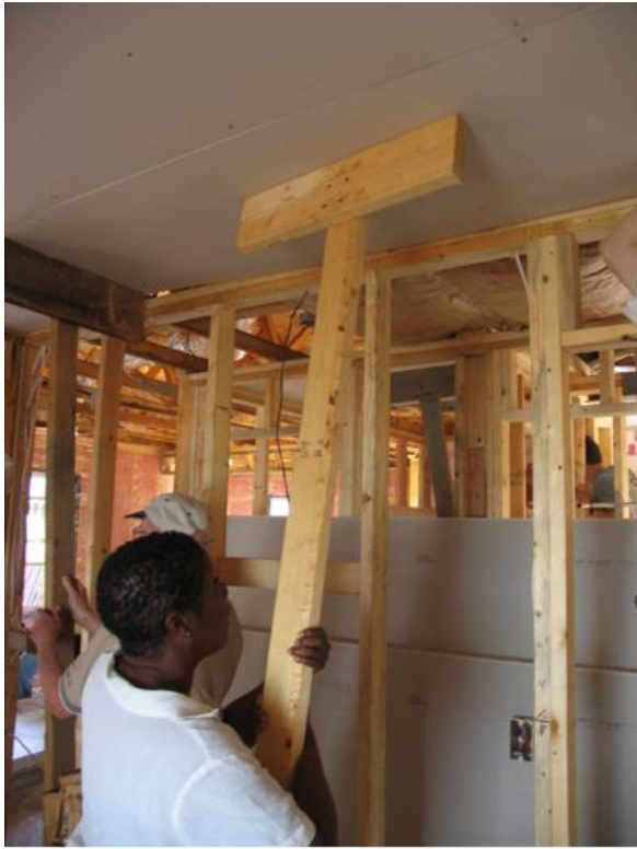
Place preachers perpendicular to trusses. Keep a hand on them at all times. They are top heavy and dangerous.
