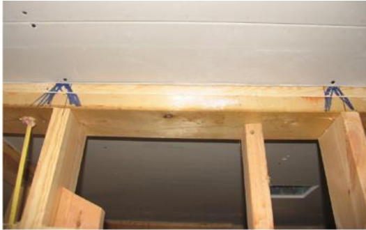
Trusses were marked on interior walls. (Hurricane clips will show trusses on exterior walls.)
