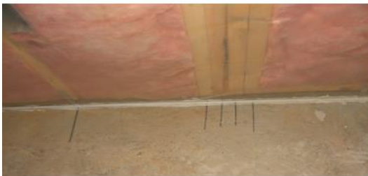
Mark all studs on floor
