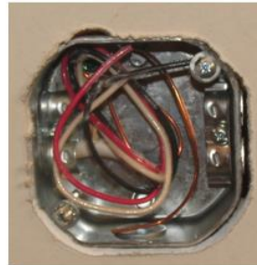
A good cut out around this light fixture.
