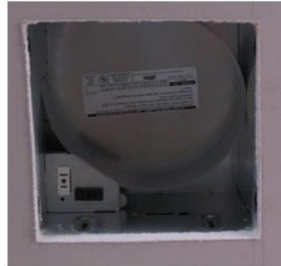
A good cut out around the vent.
