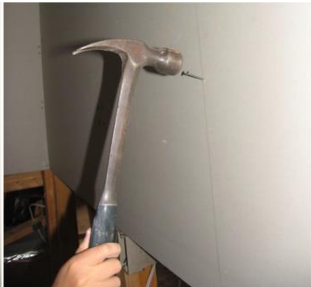
This nail is being driven in crooked and will break the paper. The hammer head will also break the paper because it is not square to the board.
