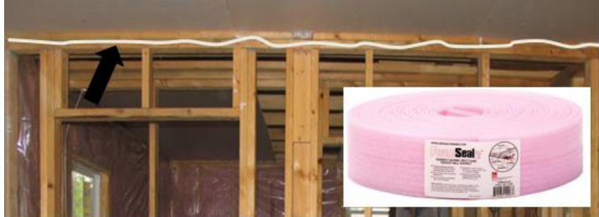
Heavy bead of caulk applied to the top plate typical all walls. Alternate Sill Sealer also shown.
