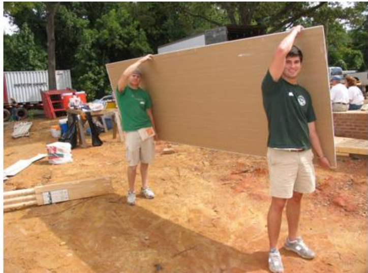
Drywall is heavy. An easy way to carry it is to keep a hand on the top and palm facing out.
