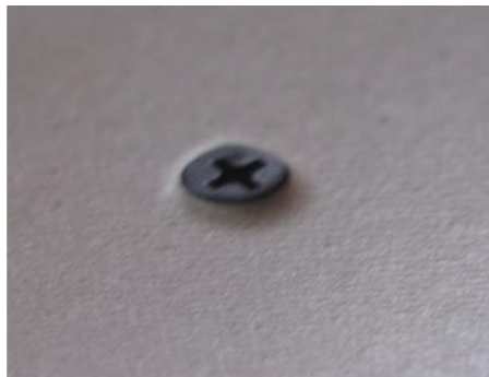
Screw Set Correctly
