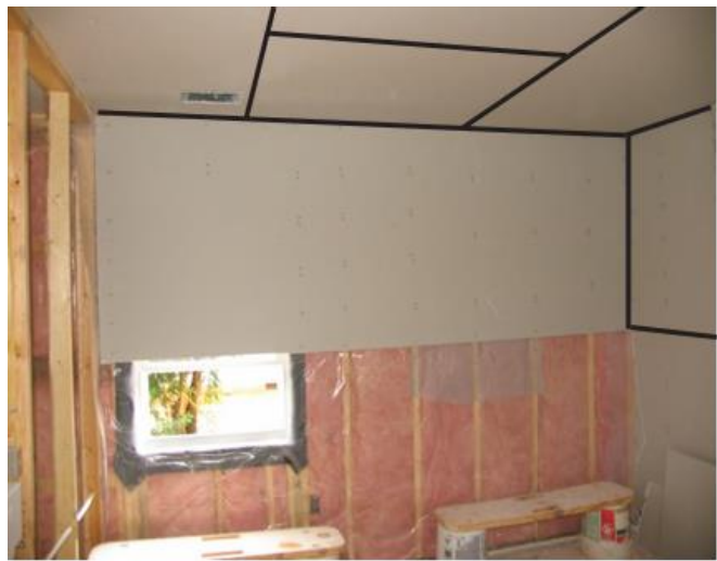
Seams are staggered at least 4'. Only factory edges are used in middle of walls or ceilings (not represented in photo).
