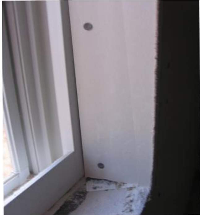
Drywall Wrap installed in window opening Normally Installed with Drywall Screws
