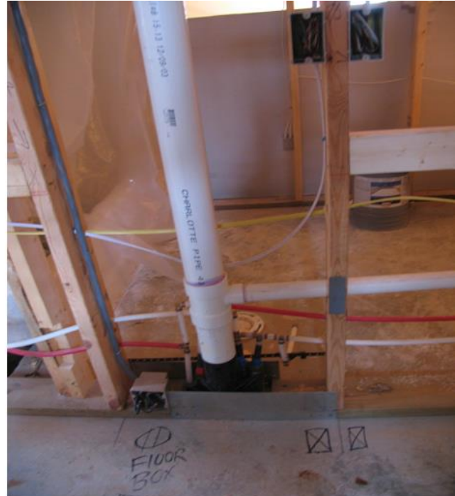
Floor is marked for outlets and range outlet. After drywall is complete, it will be easy to see if any electrical devices were missed. Notice metal plate that protects plumbing from screws.
