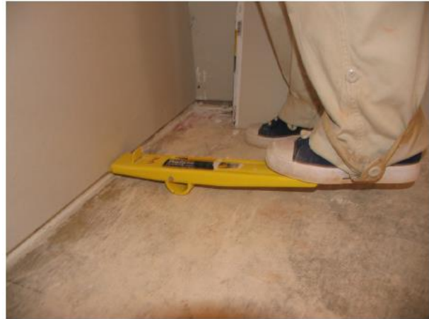
Drywall lifters raise lower panel tight to upper panel. Baseboard will hide the gap left at the floor.
