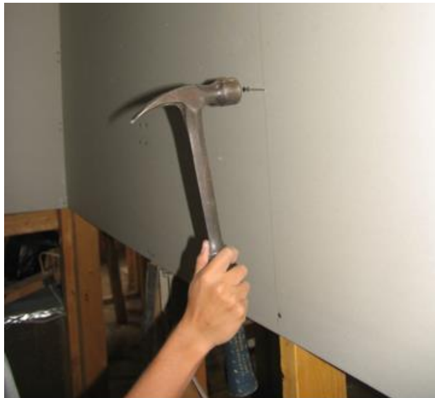
Nail being driven in straight.
