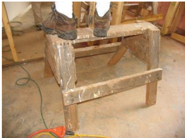
Drywall benches are easier to use than ladders.
