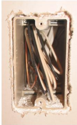
This cut is within the 1/8" tolerance.
